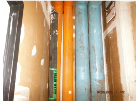
Photo 3. Asbestos-containing joint compound associated with drywall ceilings and walls are located in various rooms of the structure.
