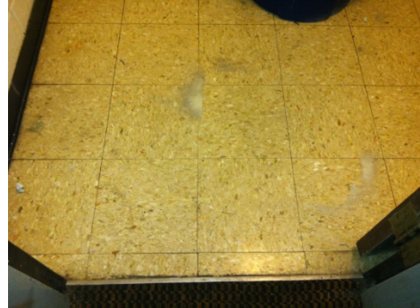
Photo 9. Asbestos-containing white overspray material was observed above the suspended ceiling tile system in the front lobby section of the building.
