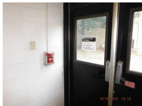
Photo 14. Asbestos-containing white interior door caulking was observed to be associated with the first floor exit doors.
